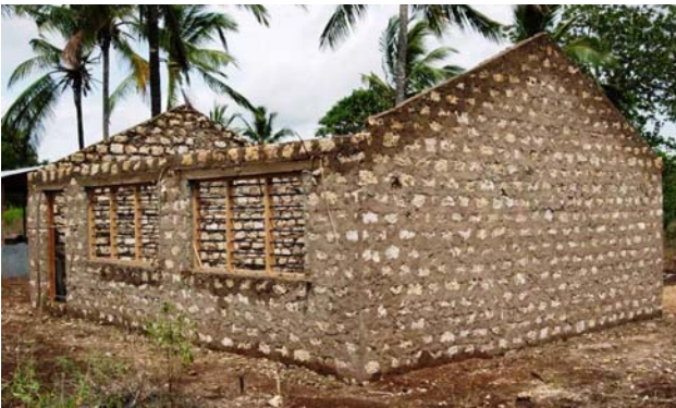
Ngoloko Village: New ECD Center Under Construction
